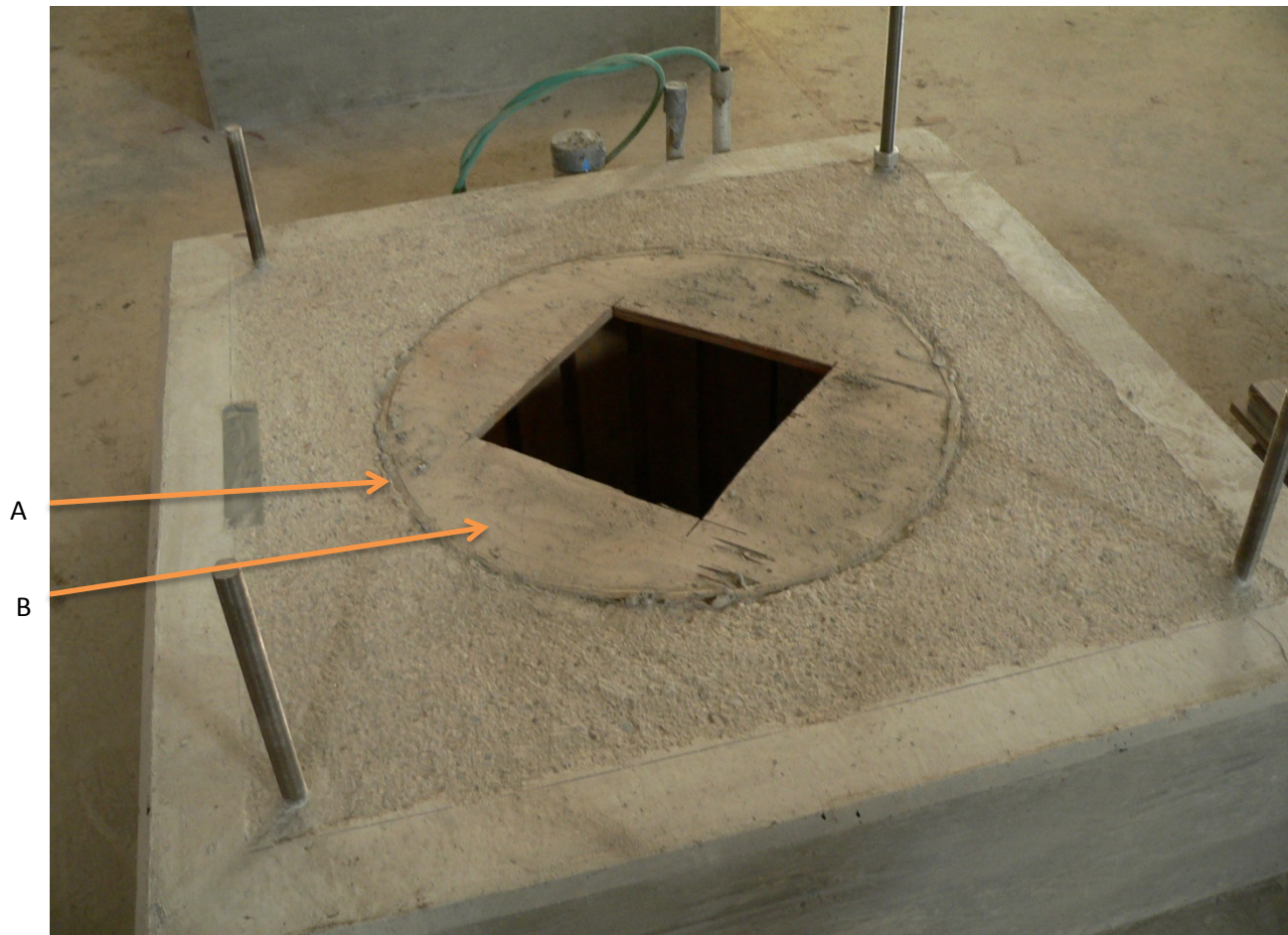
Figure 3 – Concrete pump base
