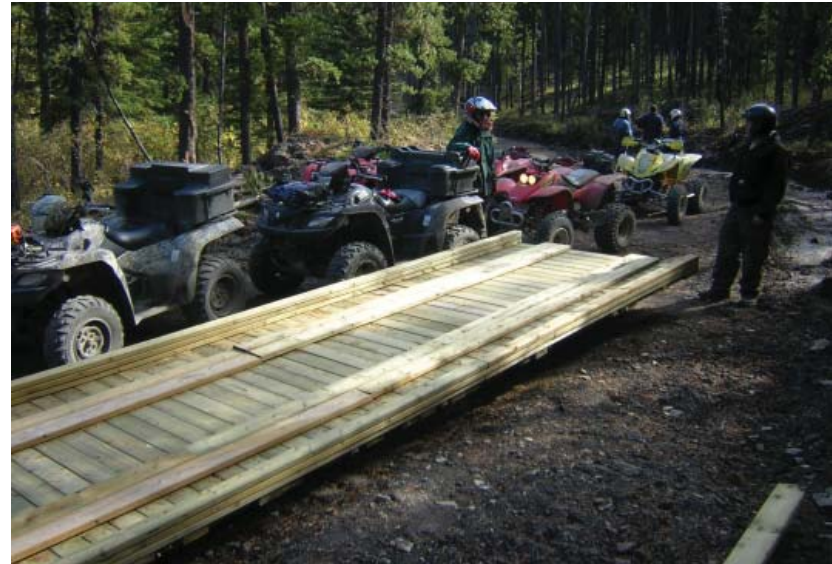
An example of a temporary portable wood bridge, also known as a 'puncheon'.
