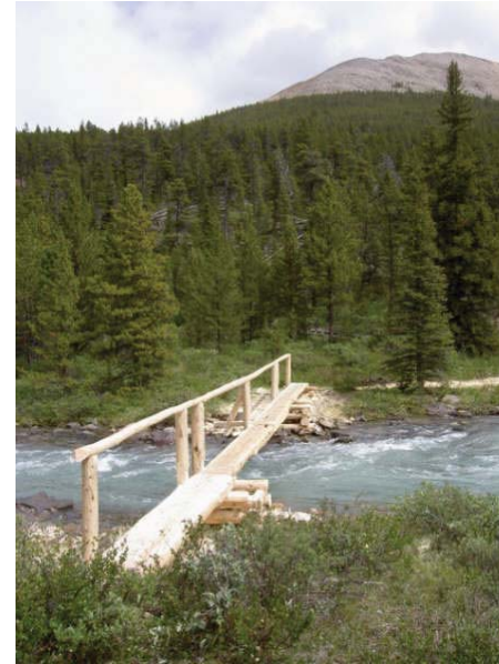
An example of a temporary log bridge.
