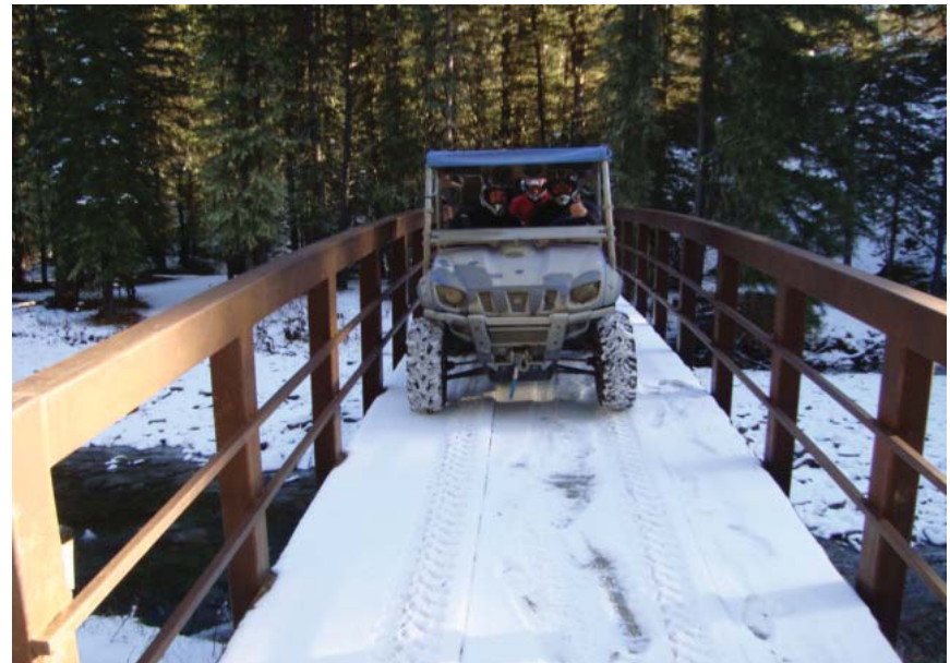
An example of a well built, structurally sound, permanent bridge crossing.
