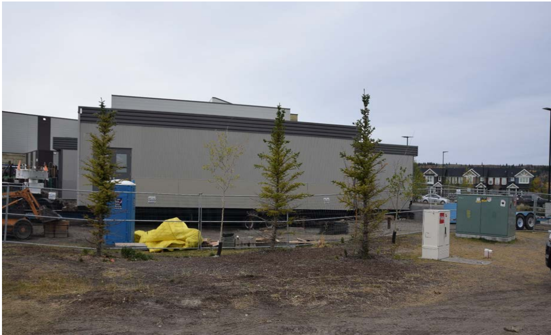
Figure 2. Side view of the portable classroom that was being moved into place at the time of the incident.
