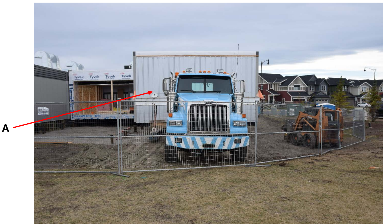
Figure 1. The truck and portable classroom that were being moved into place at the time of the incident.
