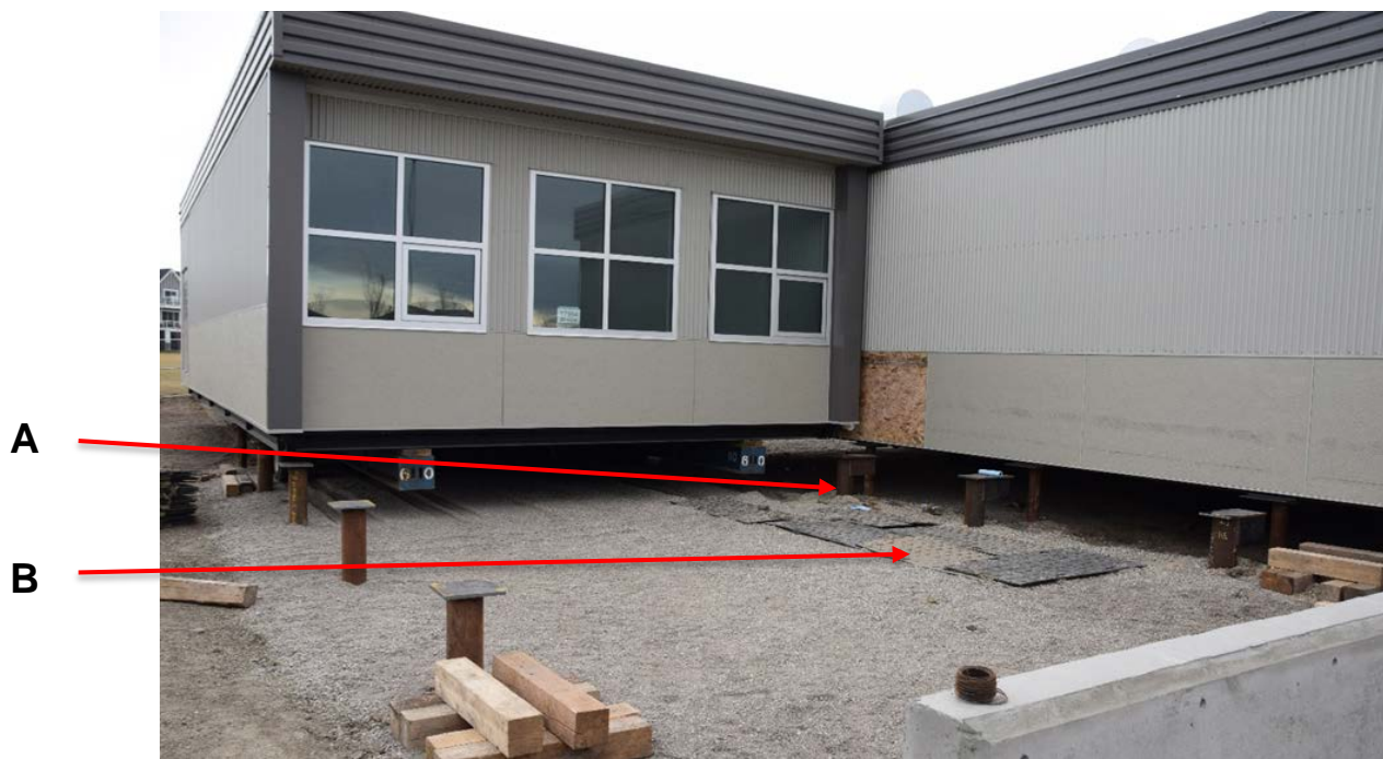
Figure 3. View of the back end of the portable classroom. This location of the portable classroom is not in situ, as the flatbed trailer was moved to extricate Worker 1. At the time of the incident, the portable classroom would have been further back.
