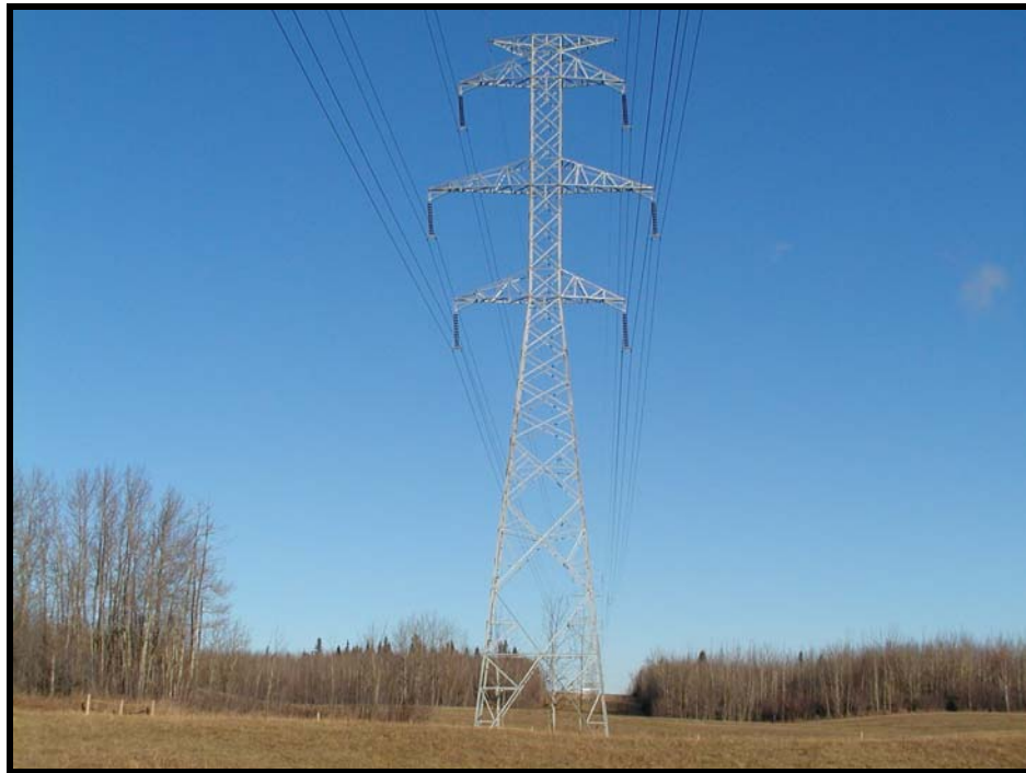
240 kV Double Circuit Tower – 4.08 m x 5.27 m.
