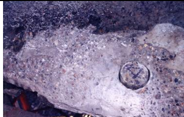
Corrosion repairs to strands may be addressed by external post tensioning. Above, corbel block.
