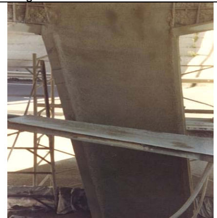
Prequalified contractors and quality inspection can produce excellent repairs.
