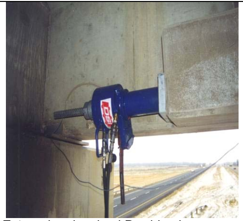
External, galvanized Dywidag bars are post tensioned – strand corrosion repair.
