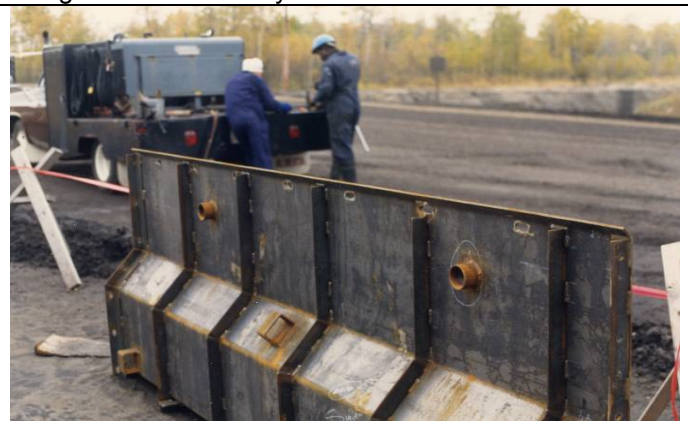
Showing steel form fabrication for recasting girder leg section.
