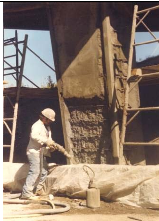
Shotcrete repairs performed to restore the pier shaft.
