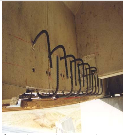
Corrosion repairs to strands may be addressed by external post tensioning. Above, corbel block.
