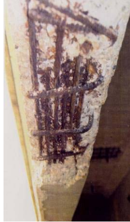
Corrosion damage to prestressing strands affects girder capacity. Investigate corrosion spall cracks to assess the extent of corrosion damage.
