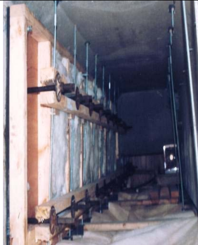
During cold weather, forms must be insulated.
