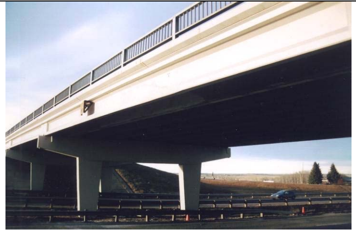
Concrete surfaces are to be finished to Class 2 rubbed finish and a matching pigmented sealer is to be applied to match existing finishes on exterior girders. Interior surfaces to receive an application of concrete sealer.
