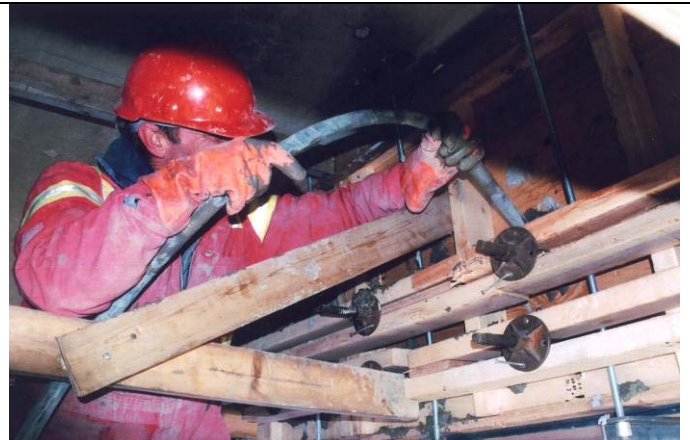
Concrete shall be vibrated to ensure consolidation around strand congestion.
