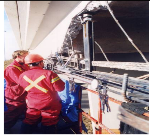
Displaced deflected strands must be positioned according to design details. Modified deflection brackets may be required to achieve design attributes.
