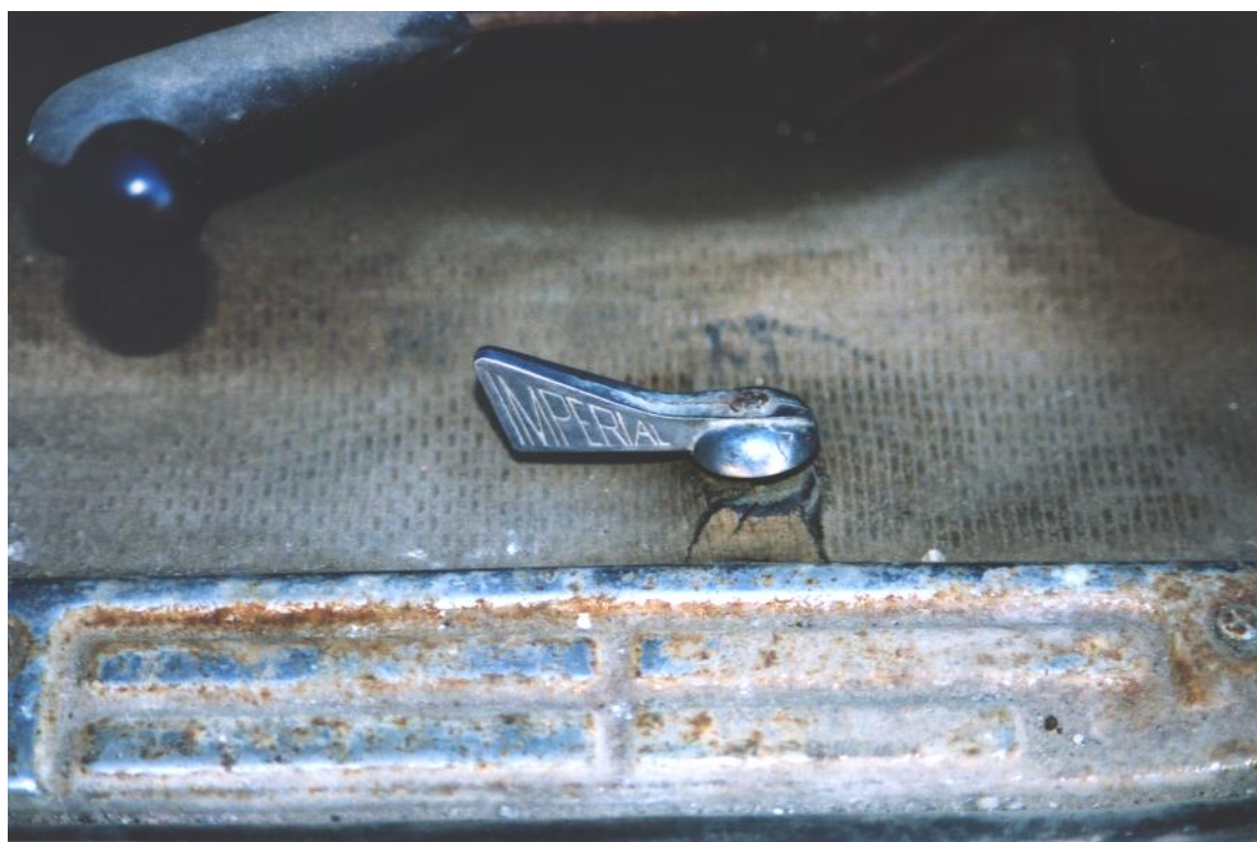
Photograph 10: Shows the 3 way valve turned to close gasoline flow from either of the two tanks.
