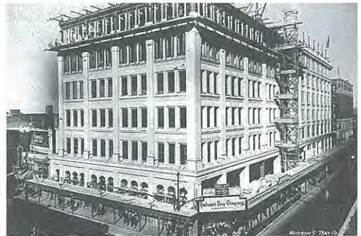
Construction of addition to the HBC Store #4, 1929. (GAINA-2037-21)
