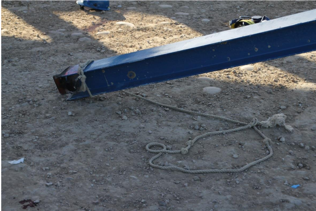
Figure 2. Photograph of I-beam with tagline attached. Photograph provided by Radium
