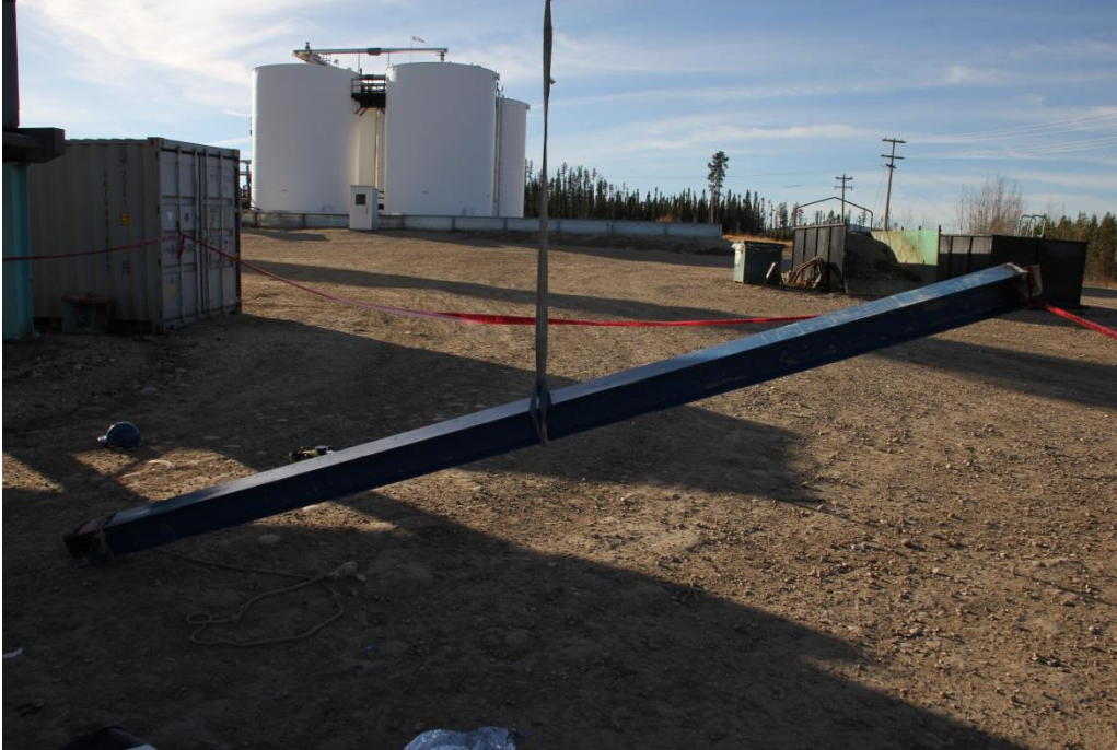
Figure 3. Photograph of I-beam suspended with sling. Photograph provided by Radium.
