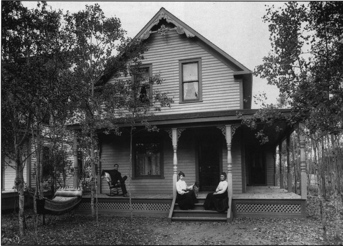
Verandahs were a bridge between the interior of the house and the outside. Photo: Provincial Archives of Alberta, Ernest Brown Collection, B4546, not dated.
