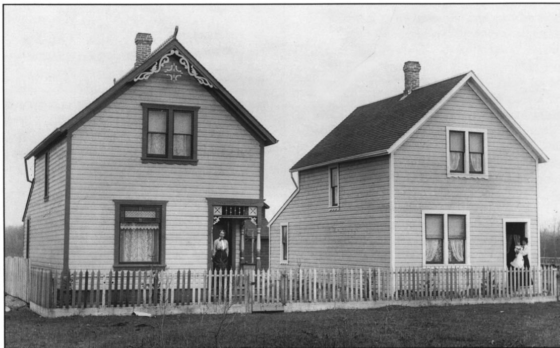
Decorative millwork, such as on the house on the left, was often mass produced and sold by lumber yards. Catalogues and advertisements contain details on such materials, as do secondary sources about the history of house design. Photo: Provincial Archives of Alberta, Ernest Brown Collection, B4582, 1903.
