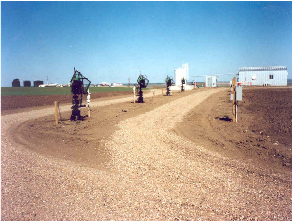
Screwjacks instead of pumpjacks
