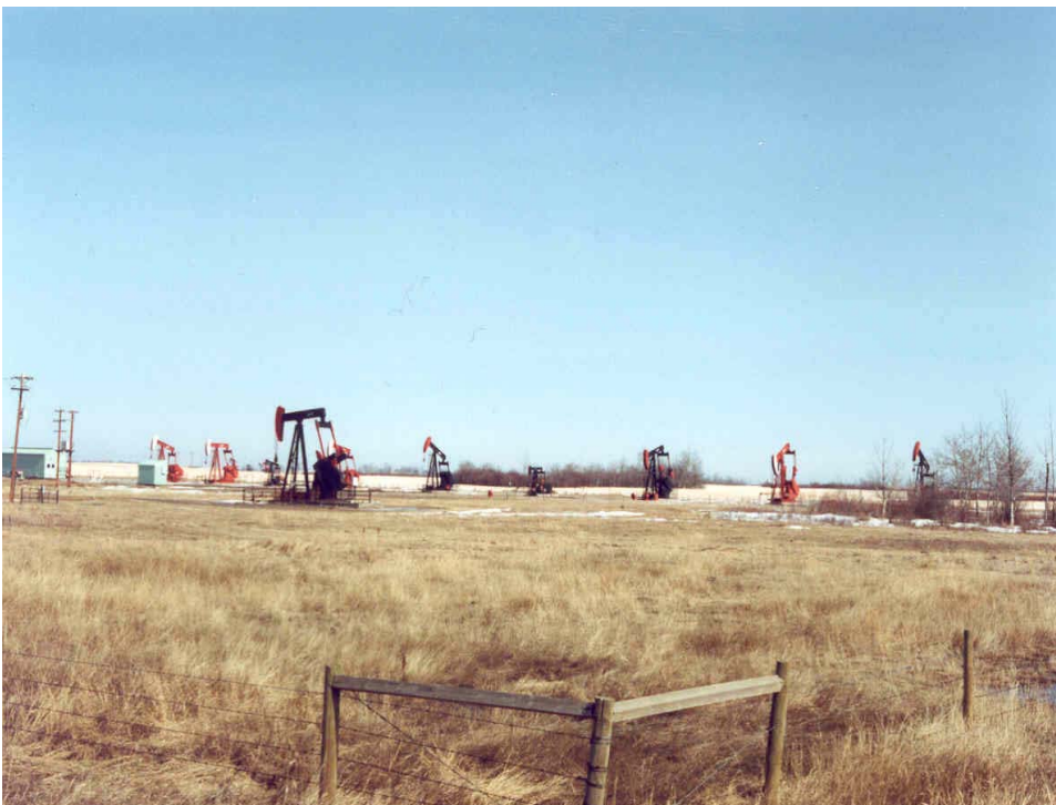
Many wells on a pad requiring downhole avoidance
