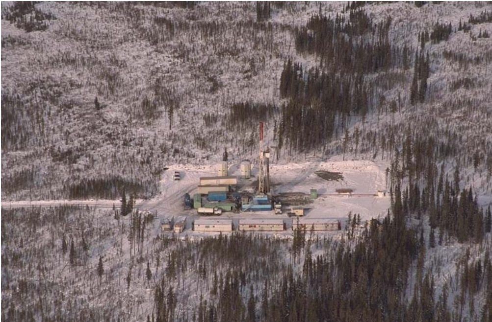
Corehole Single Drilling Rig
