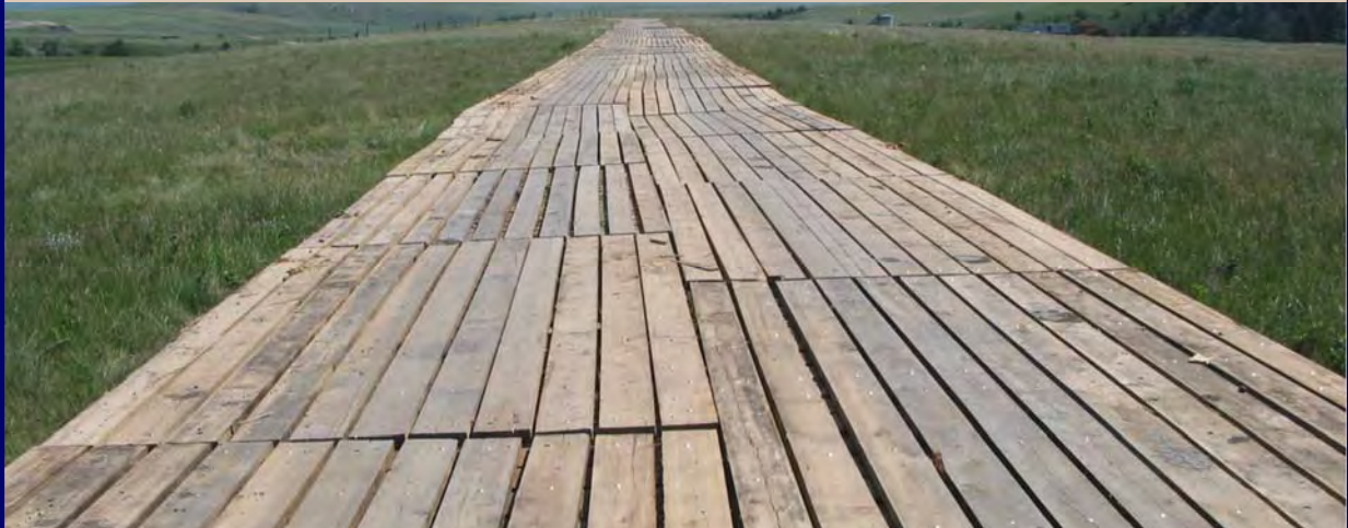
Temporary Access Using Matting to Protect Underlying Grassland.
