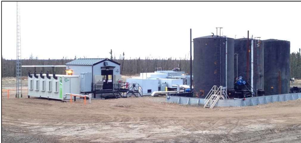
Figure 7-1: LEAD Pilot CHS Test Facility looking North
