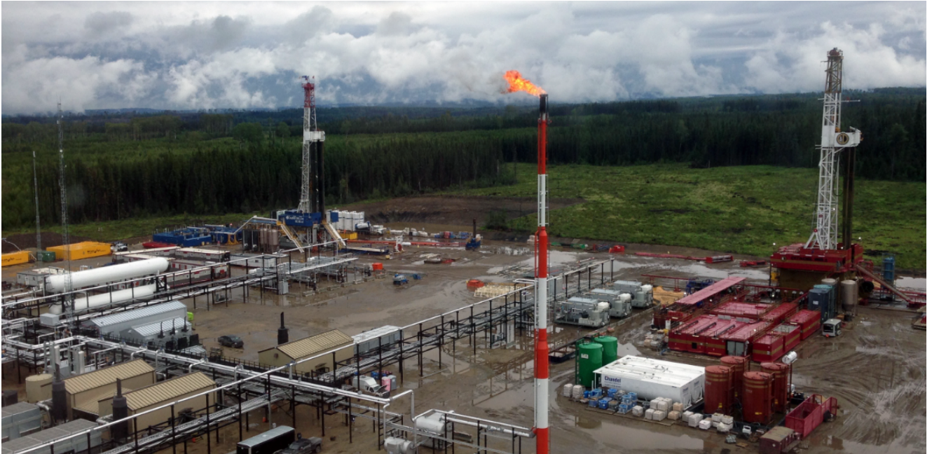
Seven Generations drilling a multi-well pad in Alberta's Montney play.
