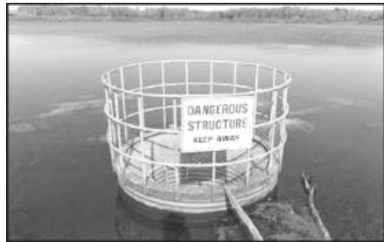
Drop Inlet Structure Figure 8 Lake
