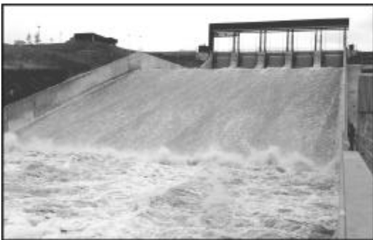
Dickson Dam Spillway
