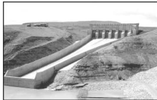
Oldman Dam Spillway
