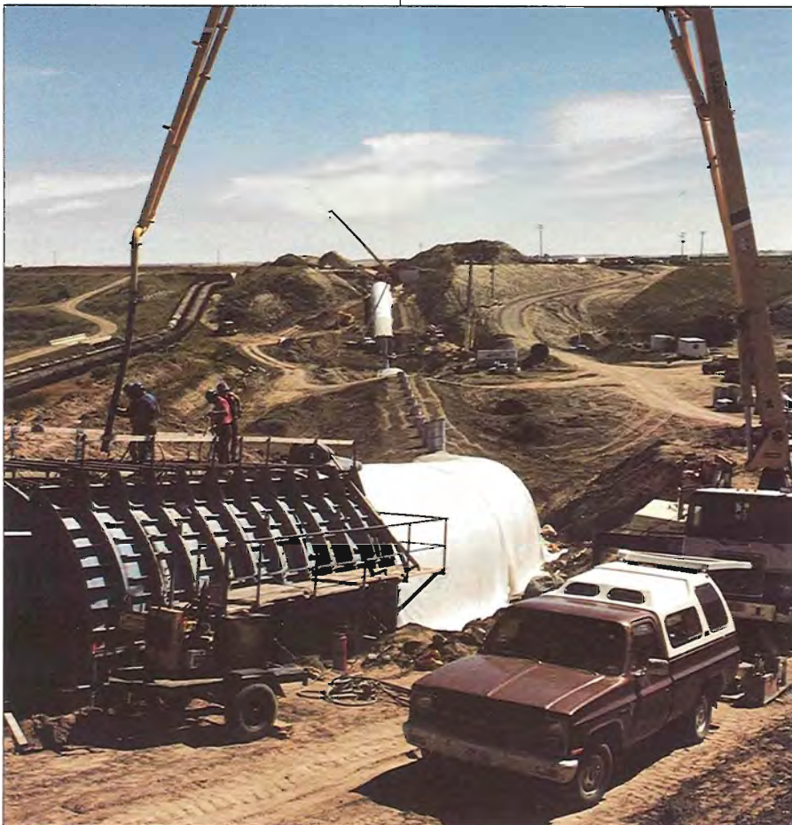
Construction of the West Arrowwood Syphon in the Carseland-Bow headworks system.
