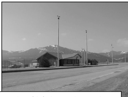
Burmis vehicle inspection station
