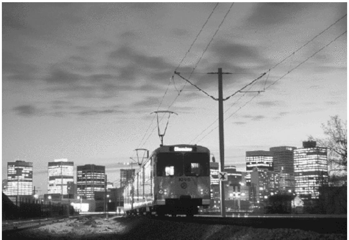
Northbound train on the Light Rail Transit line, just outside of Edmonton's downtown core.
