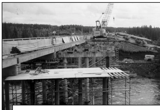
Removal of old bridge superstructure at Shunda Creek near Nordegg, Highway 11
