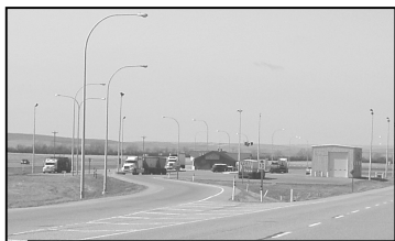
Weigh scales at Coutts Vehicle Inspection Station
