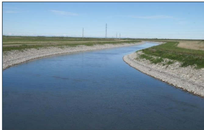
Secondary A canal in the Western Irrigation District
