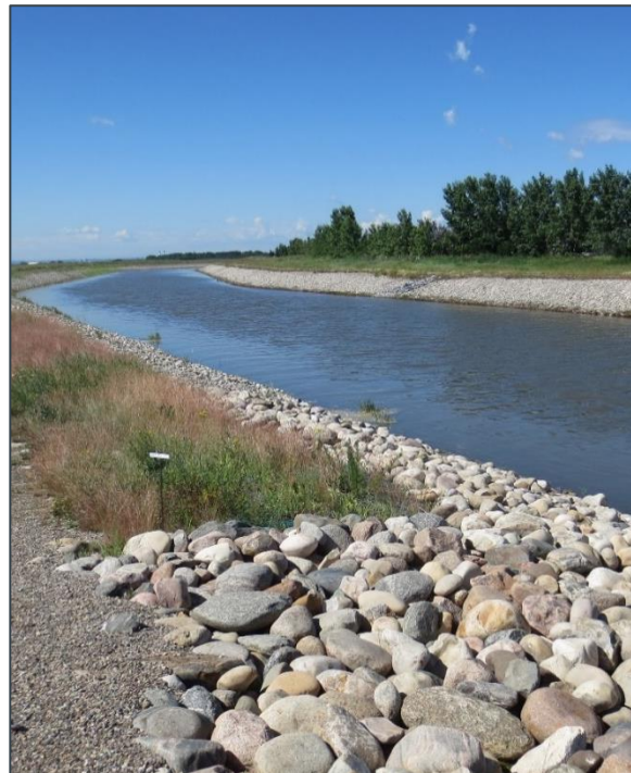
Alberta Environment and Parks canal outside Calgary carrying water diverted from the Bow River to the Western Irrigation District
