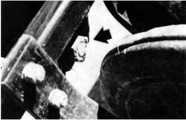
FIGURE 14. Bolt Wear on Gang Pivot Point.
