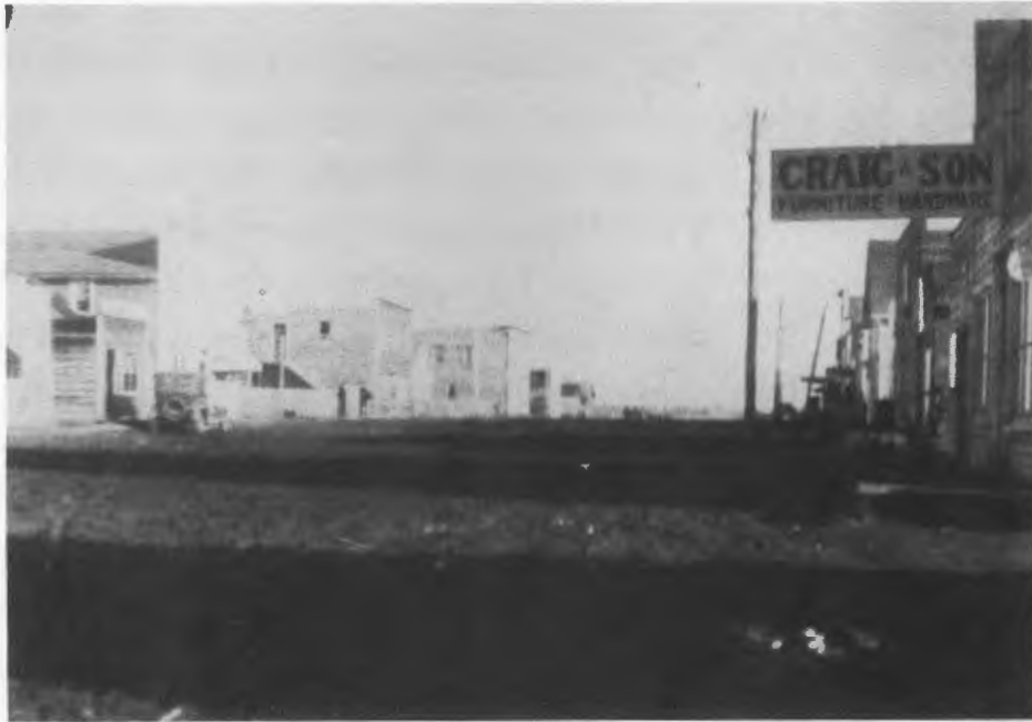
Figure 7: Buildings in the present study area, view to the northeast.
