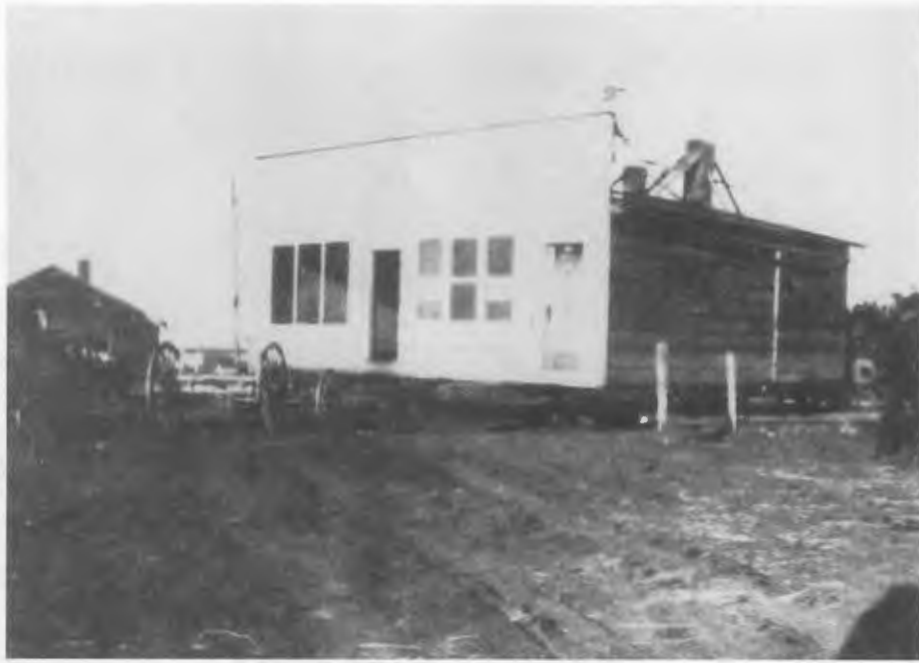
Figure 4: Building being moved from Waterhole, fall 1928.
