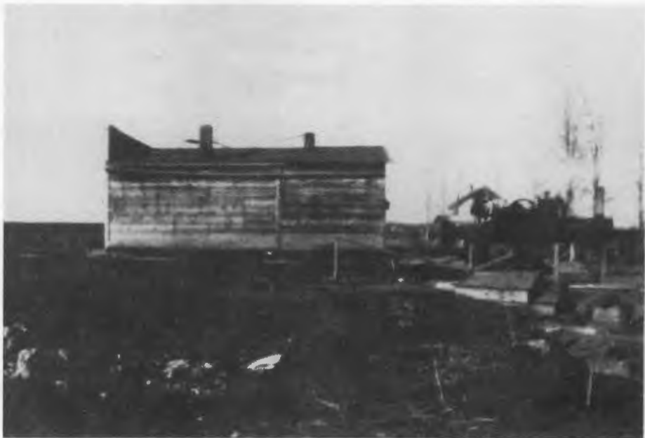
Figure 5: Building being moved from Waterhole, fall 1928.
