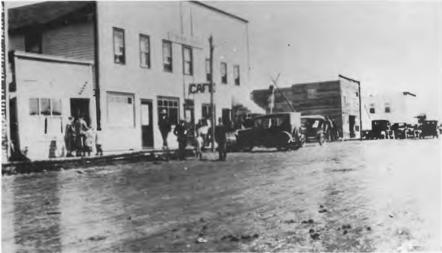
Figure 6: Buildings in the present study area, view to the northeast.
