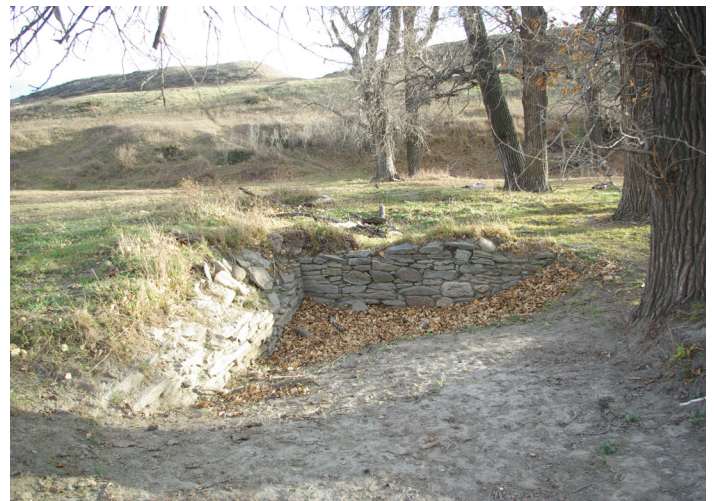
Figure 3. L-Shaped sandstone foundation, view south.
