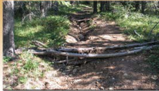
Soil erosion on the left side of the trail, due to water channelling
