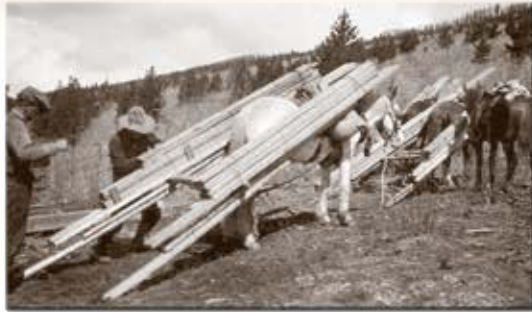
Packing lumber for construction of Coliseum Fire Lookout, 1927
