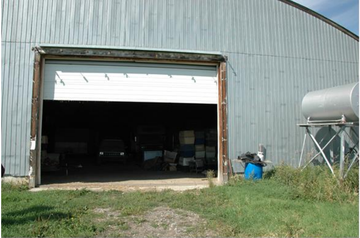
Shows the entrance to the Quonset where the incident occurred.
