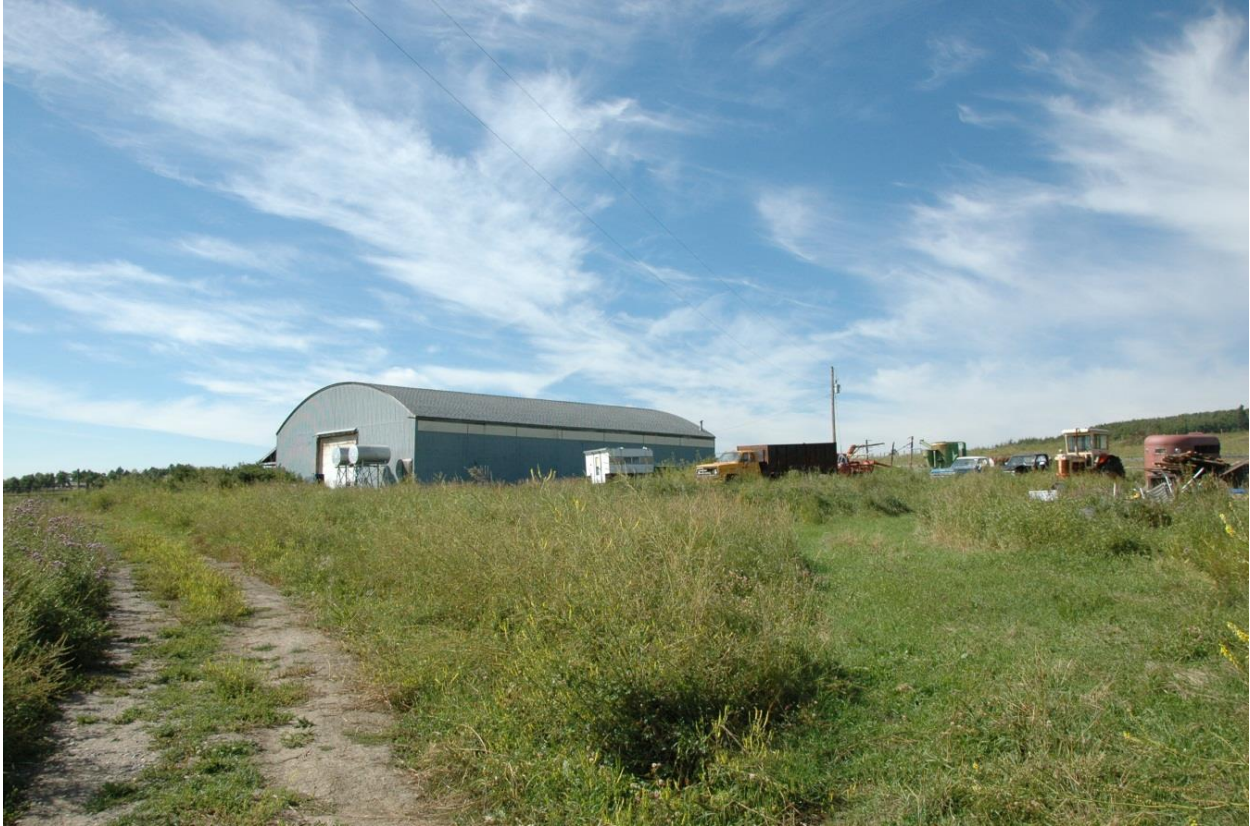
Looking Northwest, shows the Quonset where the incident occurred.
