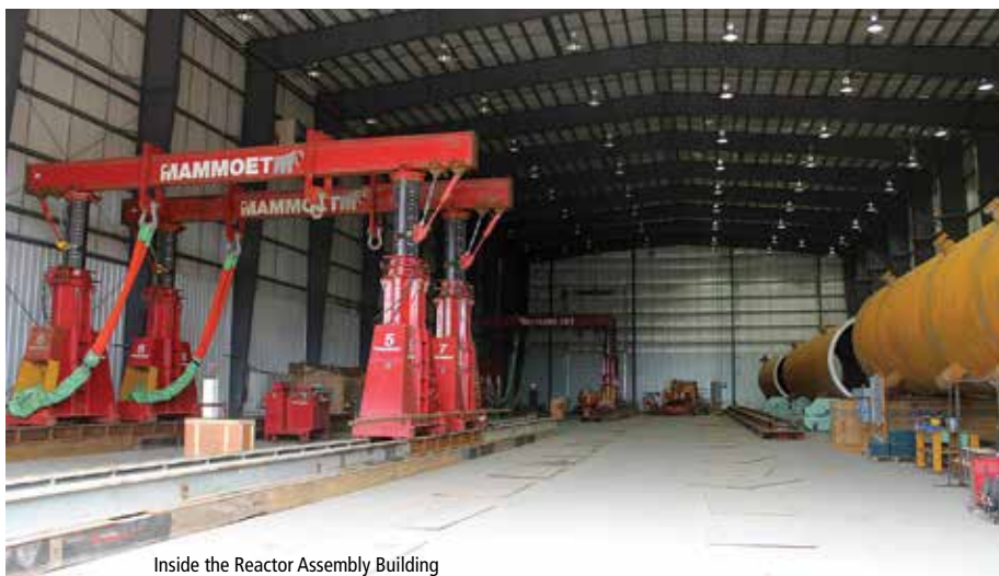
Inside the Reactor Assembly Building
