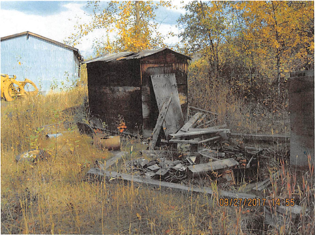
Photograph 2.f – shed containing fuel, oil and greases in the centre of the frame with garbage, debris, and refuse in the foreground and the shop with the cement floor in the background.
