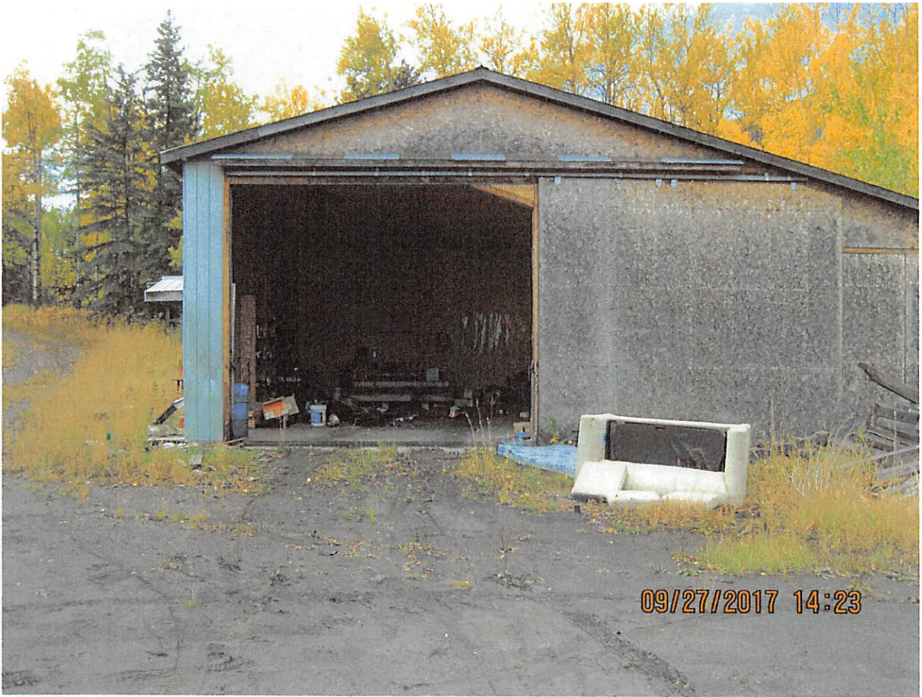
Photograph 3.b – shop and cement floor with furniture and manufactured wood products in the foreground right side of the frame. Garbage, debris, refuse and a structure can be seen to the left of the shop in the background.
