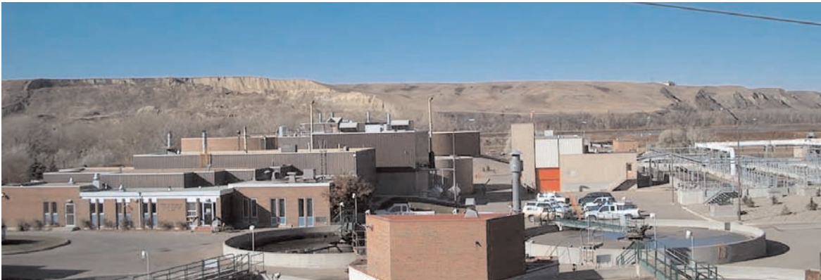
LETHBRIDGE WASTEWATER TREATMENT PLANT
