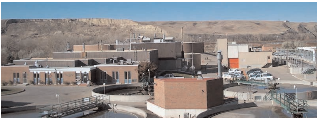
LETHBRIDGE WASTEWATER TREATMENT PLANT
