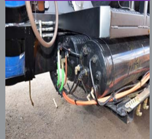
Air tank check valve
