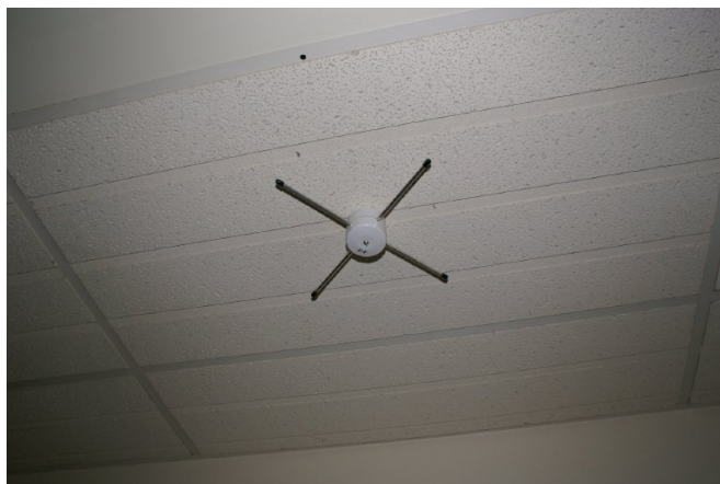
Typical emergency pendant system antenna
