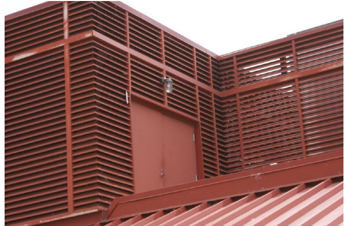
Exterior incandescent wall mount fixture.
