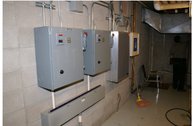
Square D magnetic motor starters
