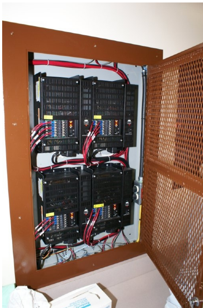
New power supplies installed in existing panels.
