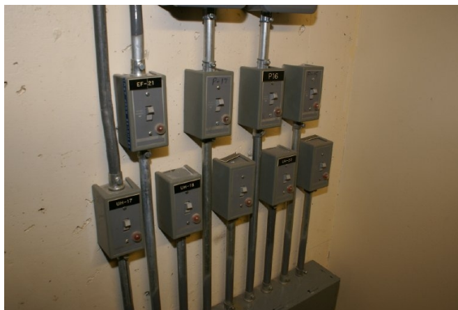
Typical manual motor starters
