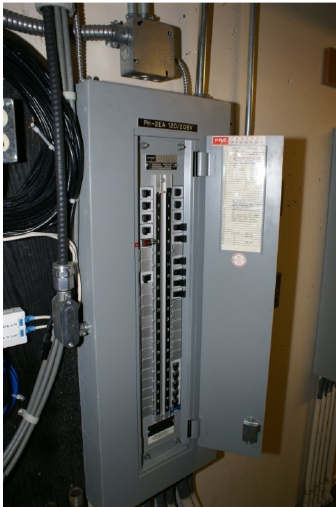
Typical 120/208V 3ph 4w branch circuit panel
