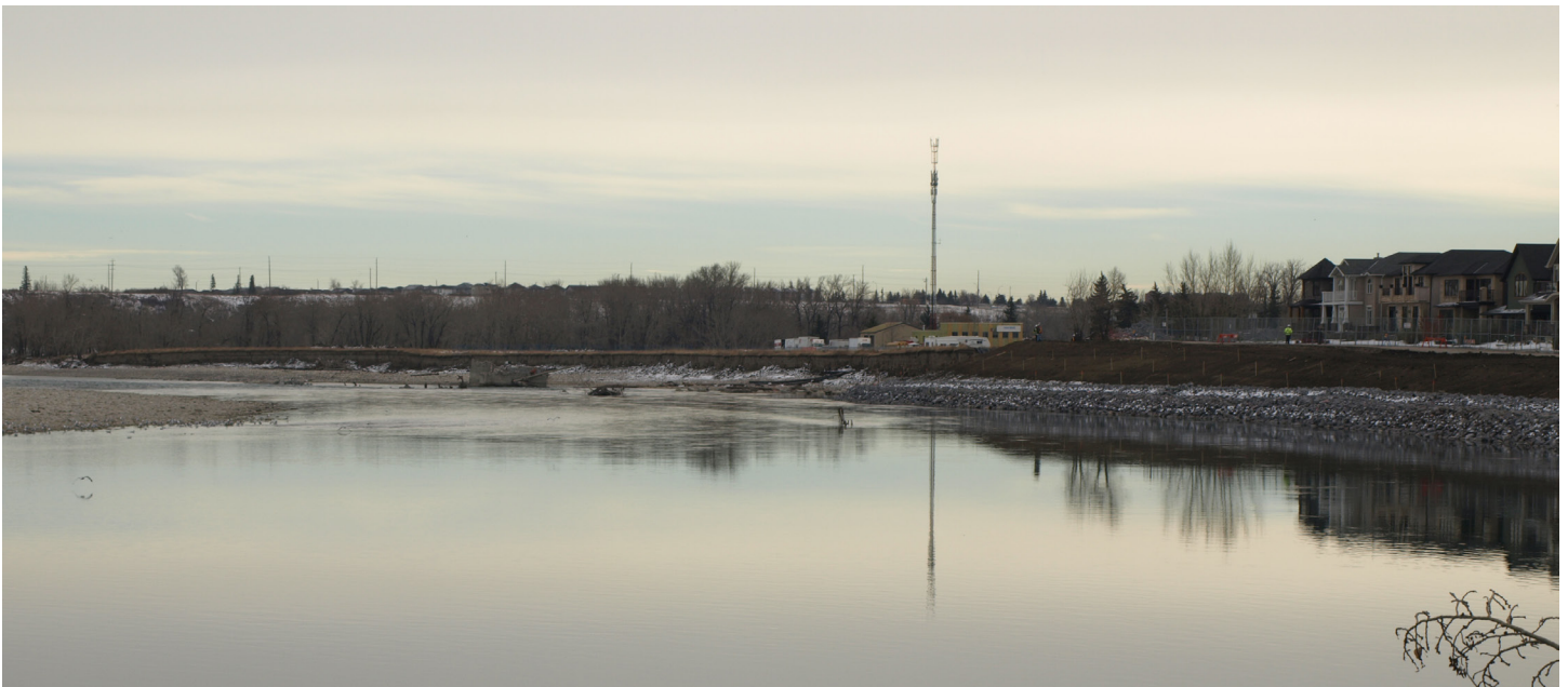
Figure 1. Example of flood damage observed at Inglewood.
