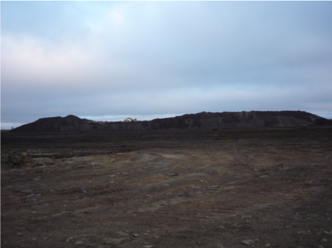
Image 12. Larger stockpile under construction.
