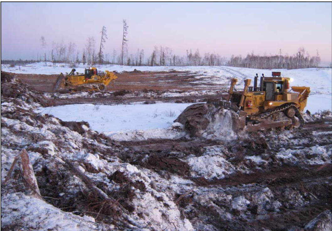
Image 11. Upland surface soil salvage of a d ecosite in winter.
