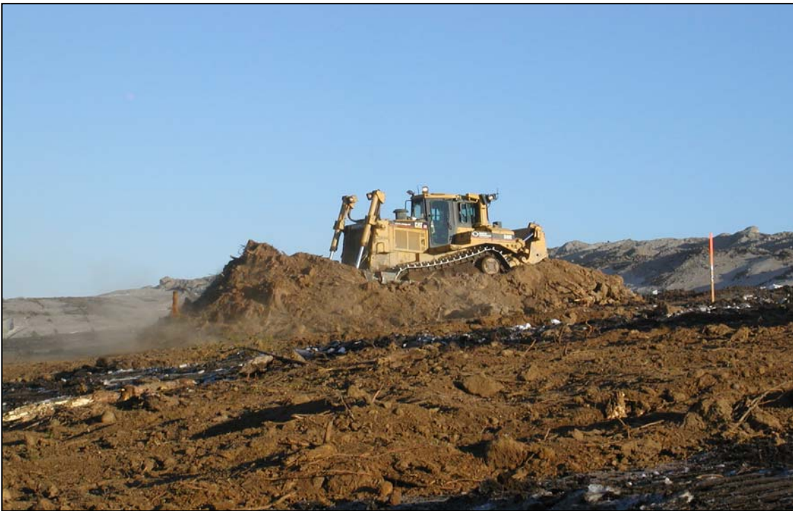
Image 16. Placement of upland surface soil from an a ecosite on a peat-mineral mix substrate.
