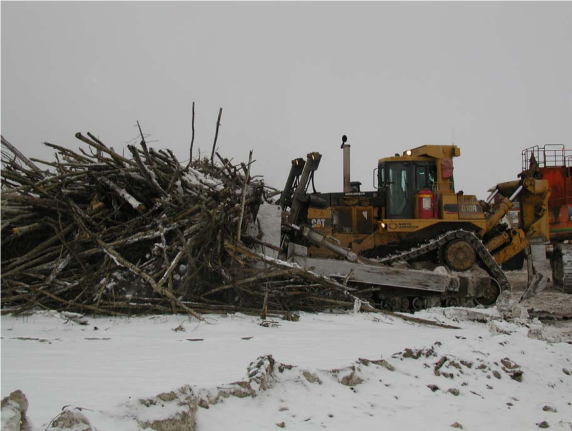
Image 8. A slash pile moved to recover the upland surface soil underneath. This is considered a best practice.
