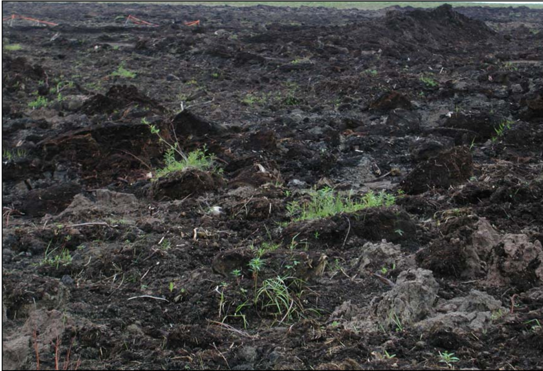
Image 18. Placement of peat-mineral mix with a rough surface early after the first growing season.
