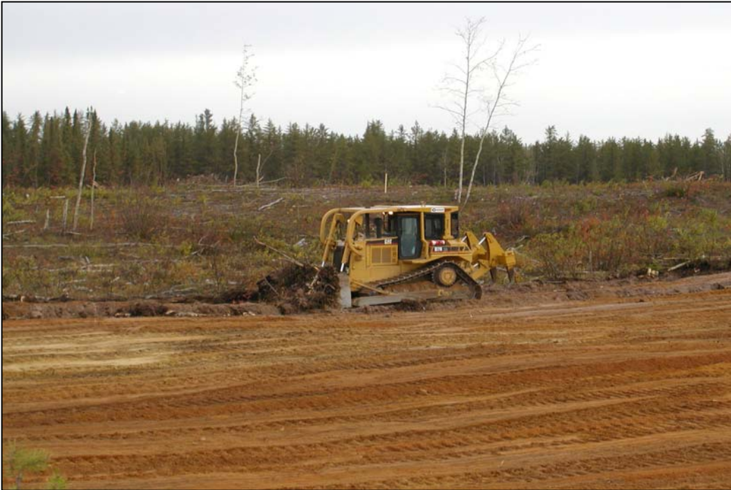
Image 10. Upland surface soil salvaged to a depth of 25 to 30 cm on a b ecosite.
