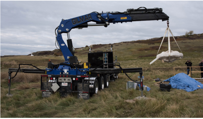
Figure 16. Lifting the jacketed feature using a cherry picker.
