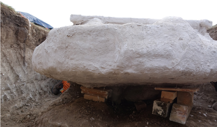
Figure 14. Detail of shoring during excavation and plastering under the feature.
