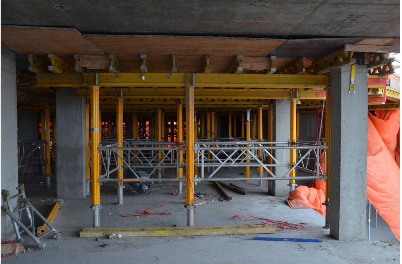
Figure 2. PERI Multiflex formwork table installed on the sixth floor.
