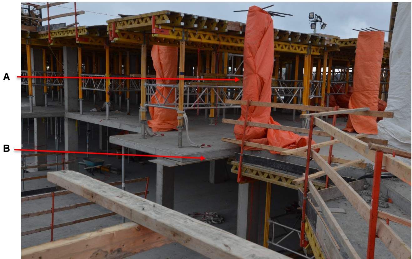
Figure 4. Incident location on the seventh floor.
