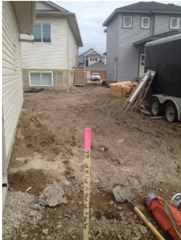
Example of temporary staking
