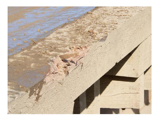
Photograph #4 Shows the impact mark made when the Foreman's truck struck the south side of the bridge.
