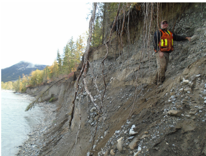
Figure 6. Debris-flow fan on the Upper Bow River (EgPs-47).
