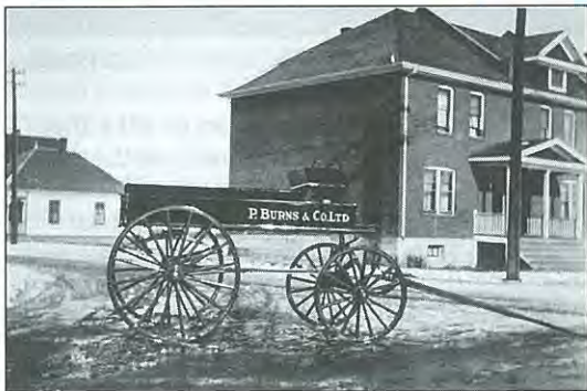
The south end of the Hamilton Apartments, ca. 1920s (GAI NA-1846-4)
