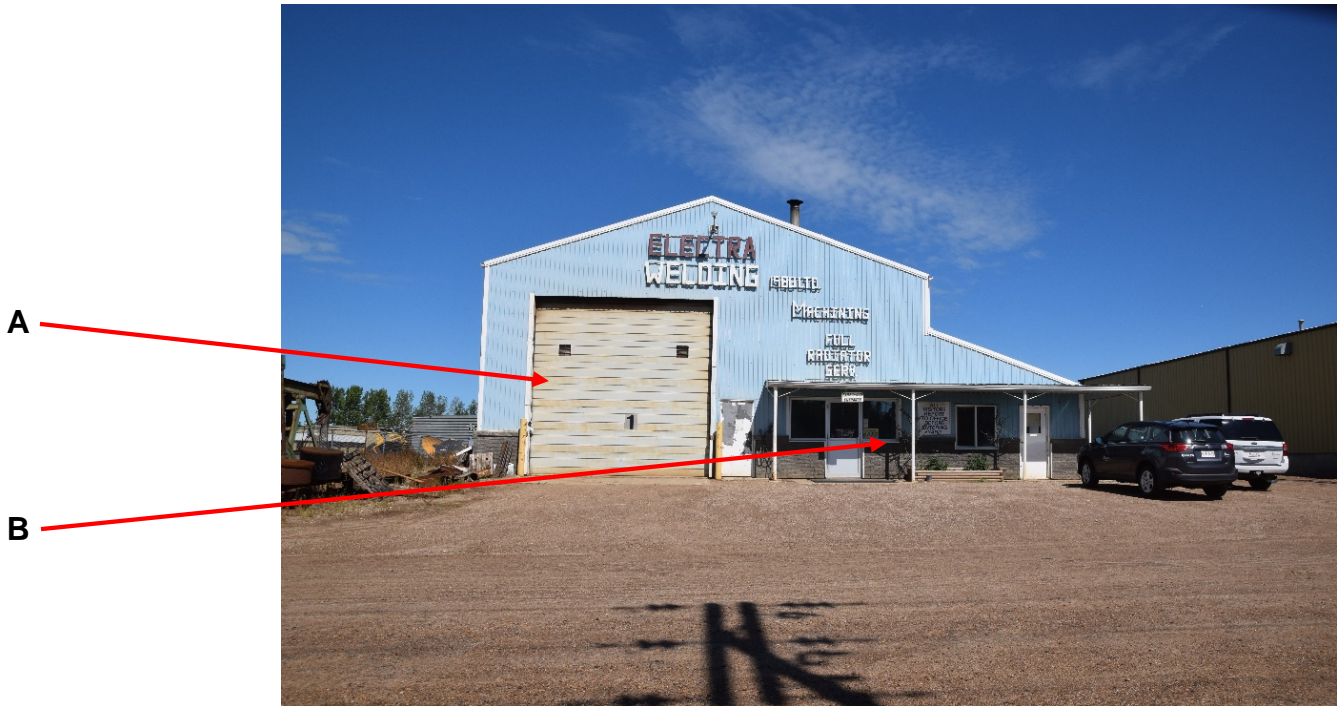
Figure 1. Electra building - south side
