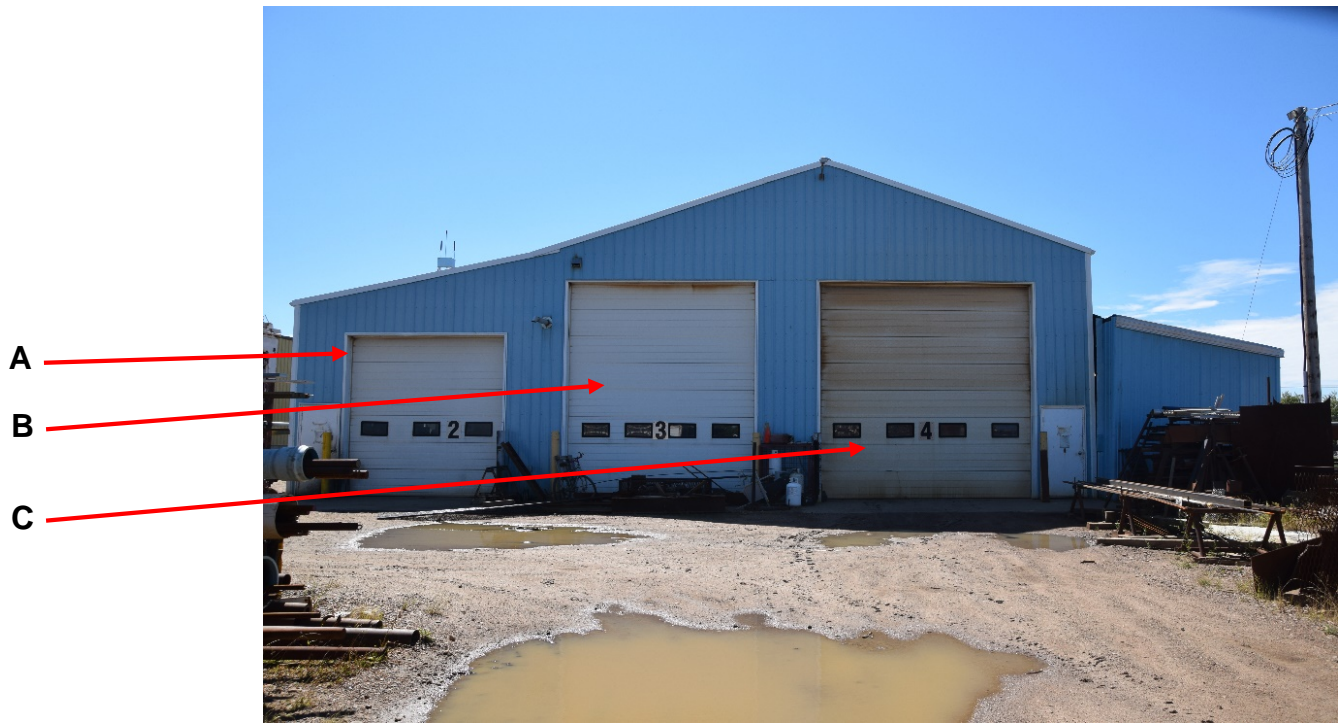
Figure 2. Electra building - north side
