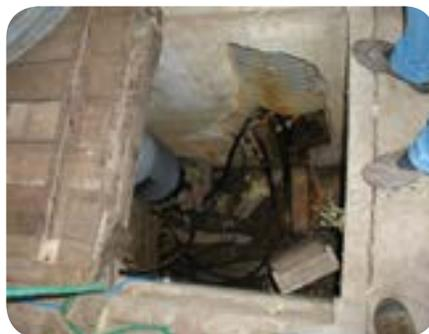
a pitless unit on the well casing and backfilling the pit. The pitless unit consists of a casing fitting and pitless adapter and provides a sanitary, water tight connection to the well casing where it connects the pump to the water distribution line (Figure 2). It is installed approximately 2 – 3 meters (6 – 10 feet) below ground level, for frost protection. Once this connection is made, the pit can be backfilled with clean clay and mounded at the ground surface.
