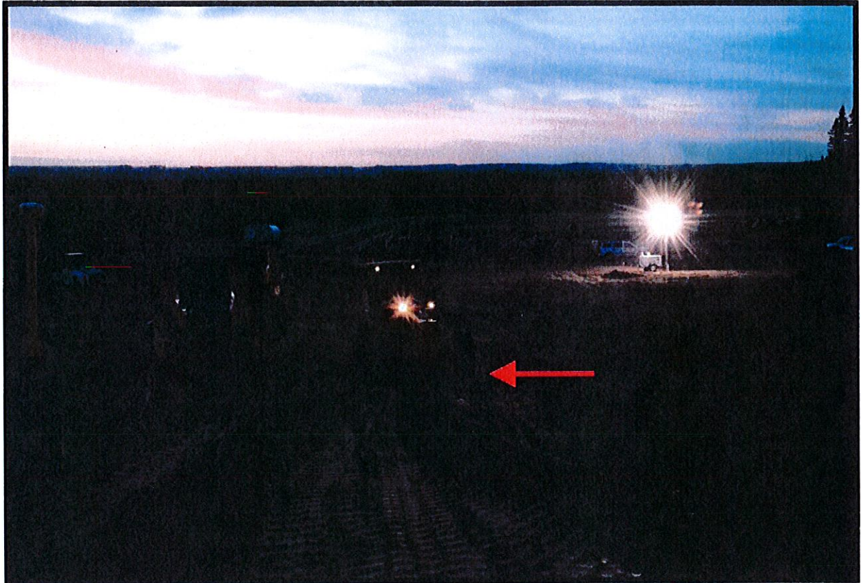
Photograph 5 – Shows an overview of the incident site with the grader lights on and the light plant operating. The arrow shows the approximate location of the incident.
