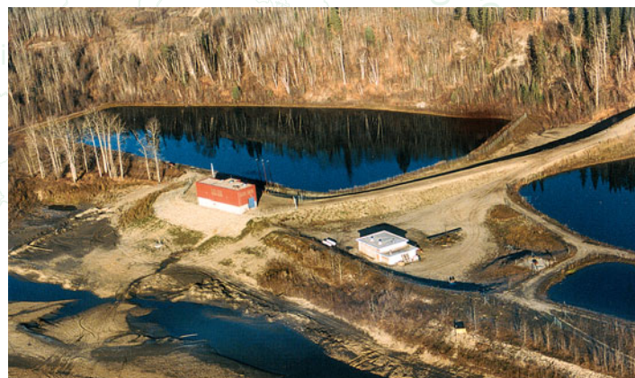
Grande Prairie's Old Water Treatment Plant and New Raw Water Pumphouse on Wapiti River (AENV)
