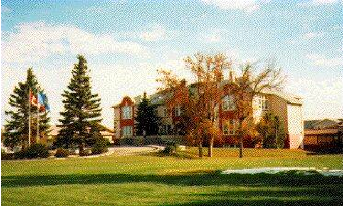
Raymond Care Centre - Main Building B0655A Raymond
