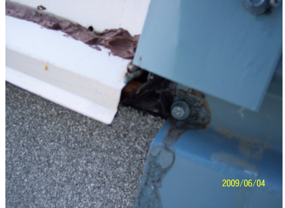
(1989) Original Building (Clerestorey of Nursing Station 148) - window sill is too short.
