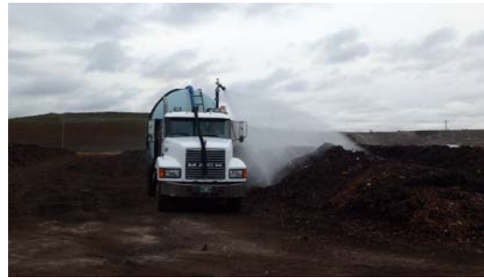
Photo 4.16. Pumping water onto a windrow with a water truck Source: CH2M
