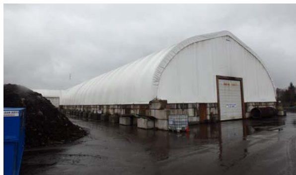
Photo 4.36. Enclosing composting activities inside a fabric-type structure can significantly reduce runoff volumes and treatment costs
