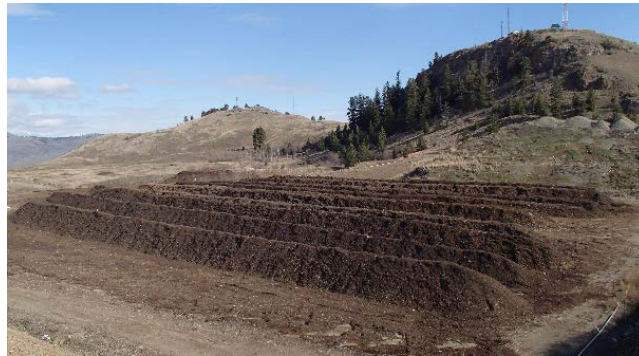
Photo 3.7. Windrow composting facility in British Columbia
