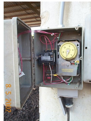
Photo 3.11. Mechanical timer used to control aeration fans
