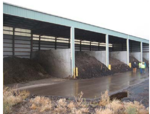
Photo 3.12. ASP system with a bunker configuration
