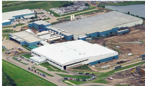
Photo 1.12. The Integrated Processing and Transfer Facility and Co-composting Facility in Edmonton is an example of a large-scale MBT system
