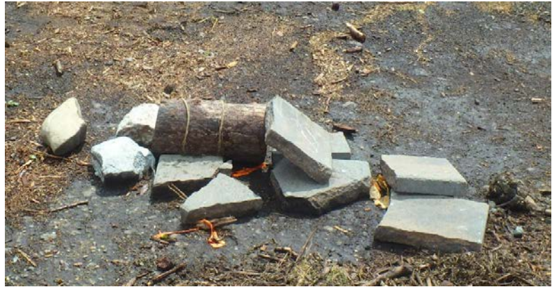
Photo 2.2. Stumps, logs, concrete and bricks can damage equipment and cause injuries Source: CH2M
