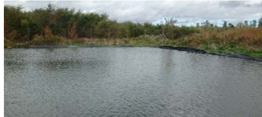
Photo 4.37. Water levels in retention ponds need to be checked regularly to prevent overflows and releases
