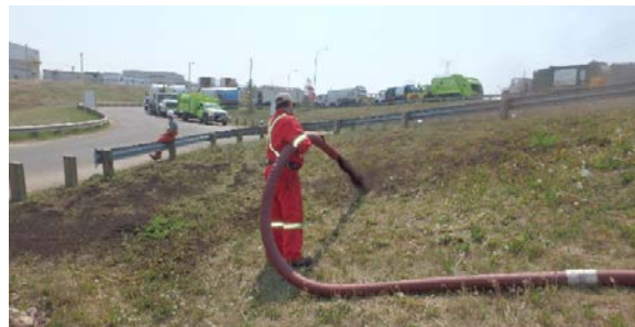
Photo 4.42. Compost being pneumatically applied to a slope from blower truck
