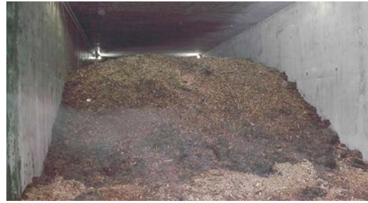
Photo 3.25. Interior view of tunnel composting system
