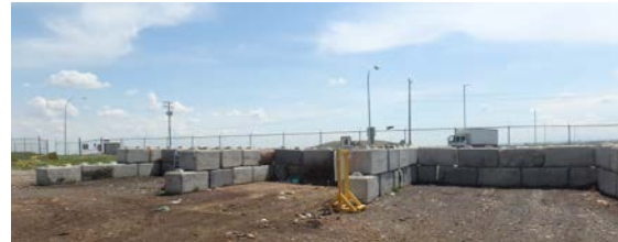
Photo 4.1. Bunkers for receiving and temporary storage of feedstocks
