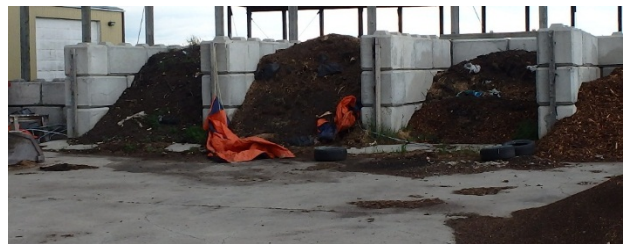
Photo 3.4. Bunker composting facility
