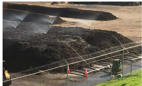
Photo 4.18. Using sprinklers to apply water to an ASP Source: CH2M
