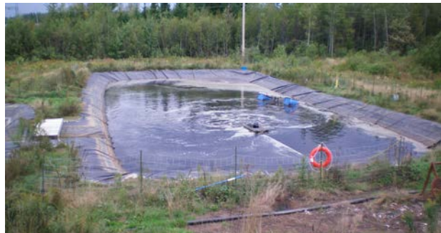
Photo 4.40. Aeration systems can be installed in retention ponds to reduce BOD and treat odours
