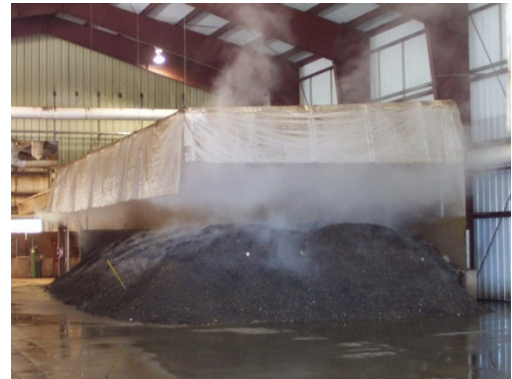
Photo 3.13. Positive ASP composting system inside at building Source: Scott Gamble
