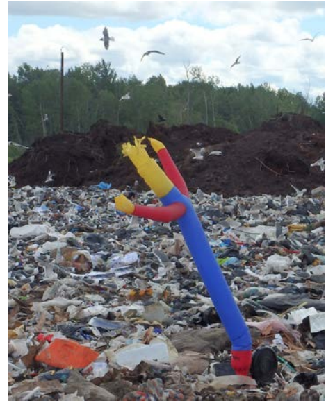
Photo 4.28. An electric “air dancer” being used to scare birds at a landfill working face.
