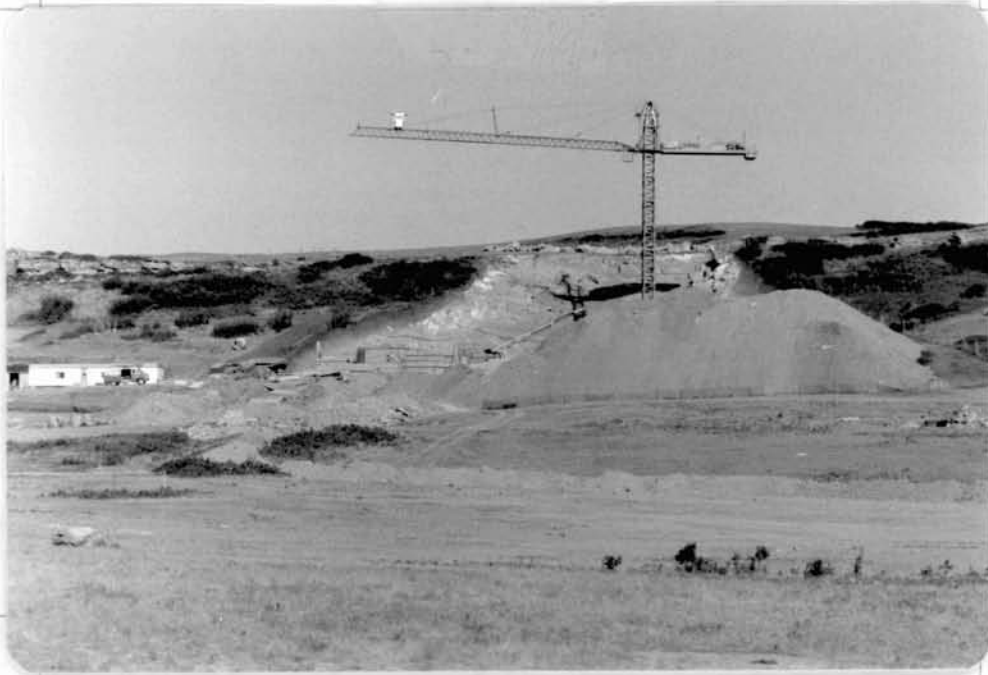
Figure 44. View of construction site.
