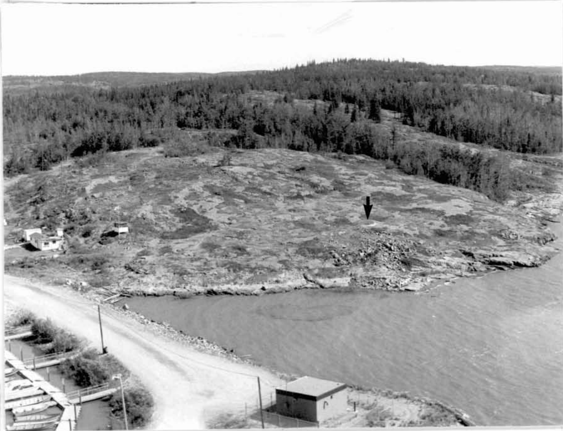
Figure 11. Oblique aerial view of powder magazine (Ie0s-4) site location, marked by arrow. View to northeast.
