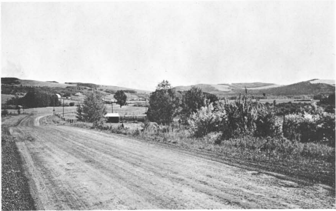
Figure 6: Looking E along SR549 west of Millarville. Building in left centre, a log barn (EcPo-18), will be destroyed by curve revision of SR549.
