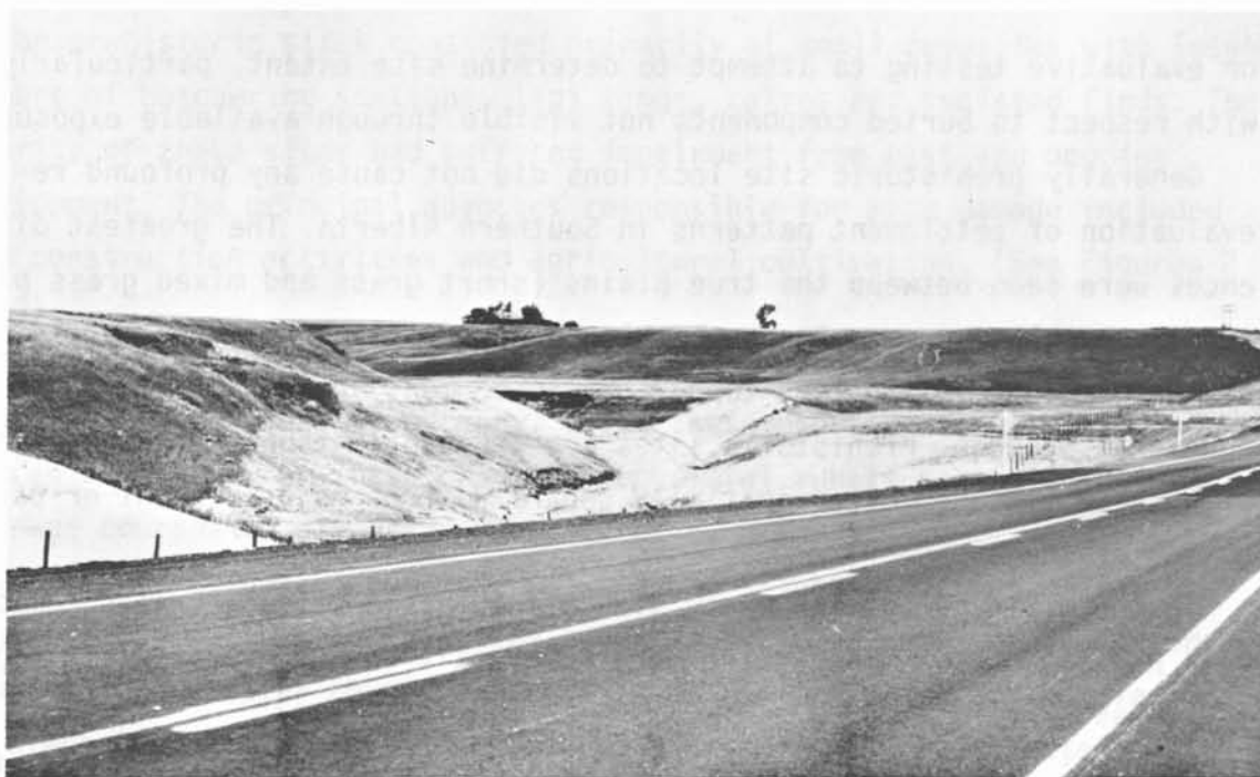
Figure 2 : Hwy. 5 Round-Up Creek Crossing. Creek diversion channel through stream terrace which destroyed much of Site DhPg-2. Looking N.
