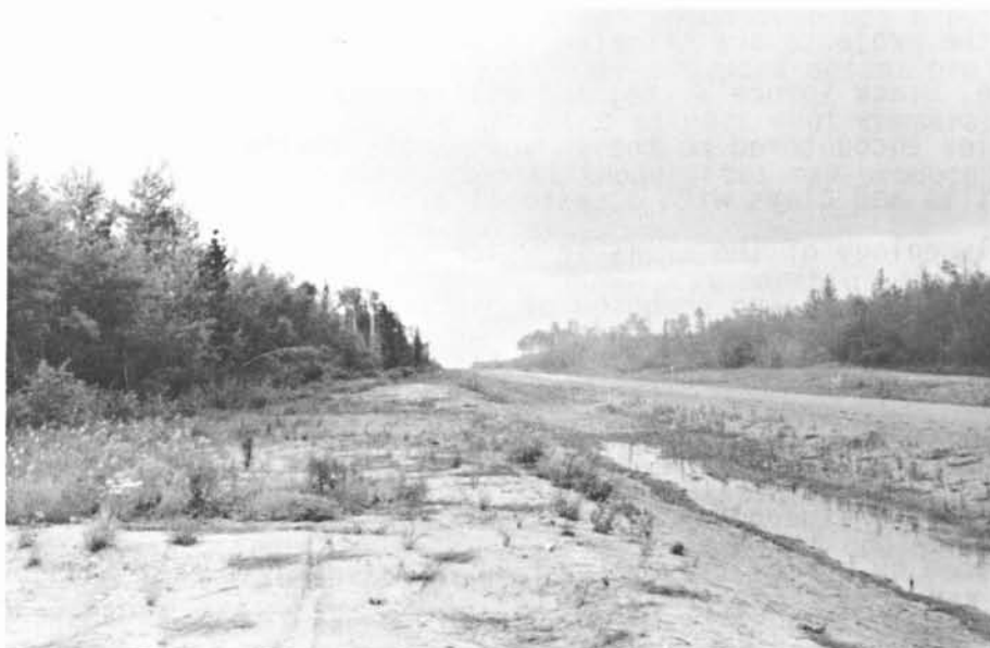
Figure 11: View north along Project 967:04 right of way showing "scalping" and removal of all upper soil horizons.
