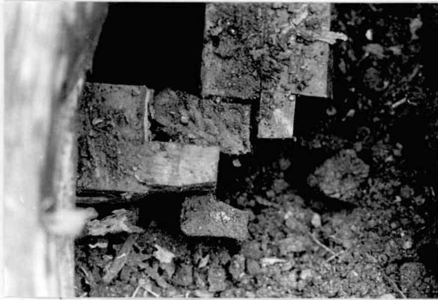
Figure 13: Exposed corner post detail at southeast corner of cellar top tier. (Historic Sites Service photograph Cat. No. R2M-1118-M).
