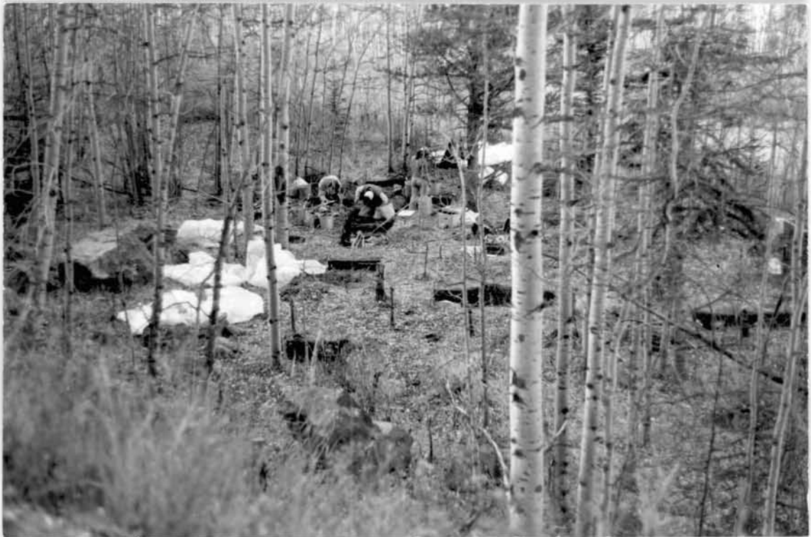
Figure 29: EfPq-6 During Excavation.
