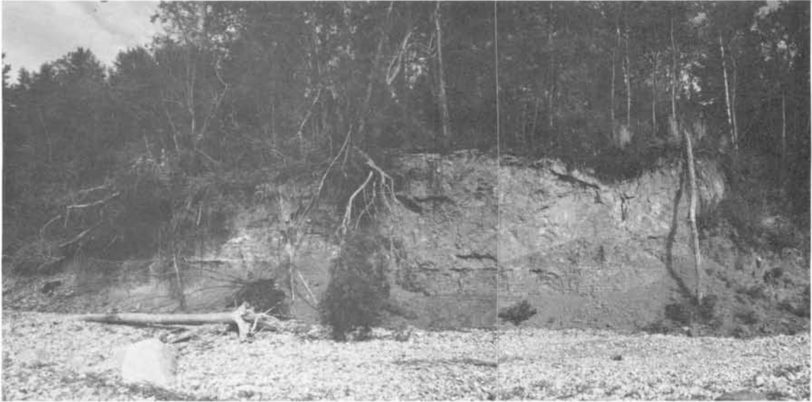
Figure 64: View of the Slump Site (GiQa-3) showing the eroding face of the exposure.
