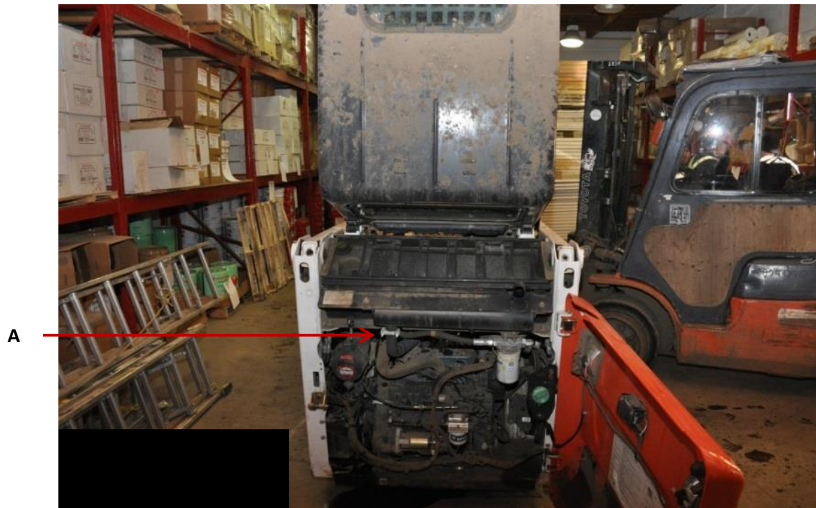
Figure 2. The opened back door to the skid-steer. A: The loosened circuit hose.
