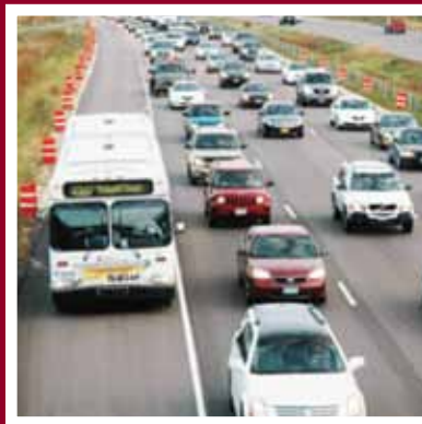
ROAD LANE REDUNDANCY One lane beyond capacity needs and dynamic shoulder lanes
