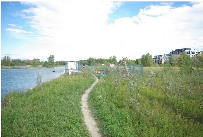
Figure 2. View north of EfPm-267, the primary excavation block is located inside the fenced area.
